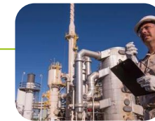
Sulfuric acid regeneration
